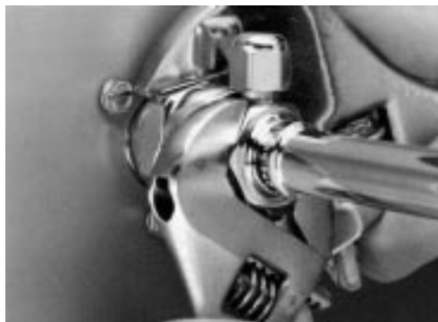
Tighten Swivel Nut
